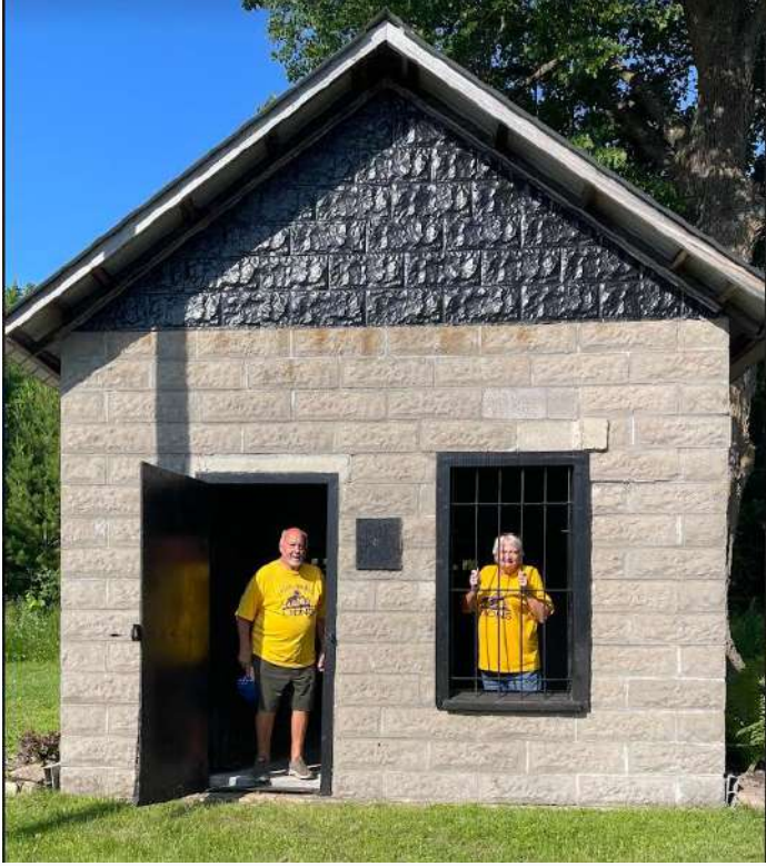
Benedict Laporte Lions Jail restoration project by Lions Keith Littis and Shelly Jacobsen worked many hours the past 3 years to restore the Laporte jail.
